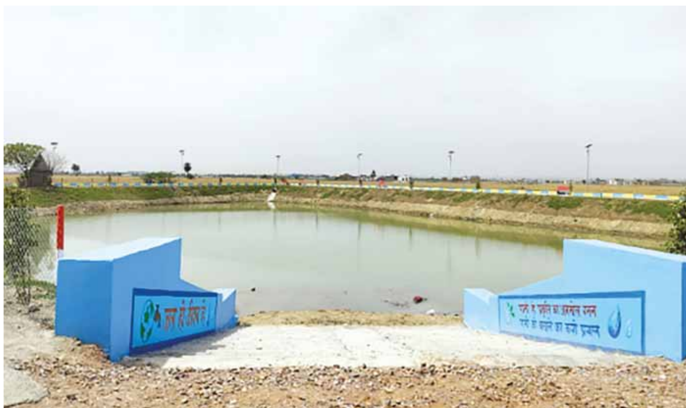
Pond rejuvenation done at Sikrona village, Faridabad
